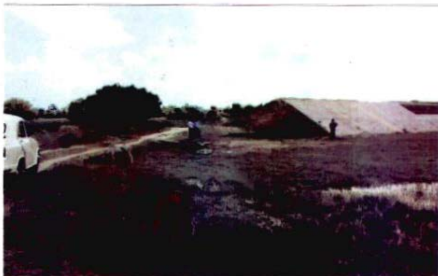
Dauk Nagar Main Canal of TBP at Ch. 63.585 where no trace of canal water was observed due to land dispute in Uttar Dinajpur District, (WEST BENGAL)
