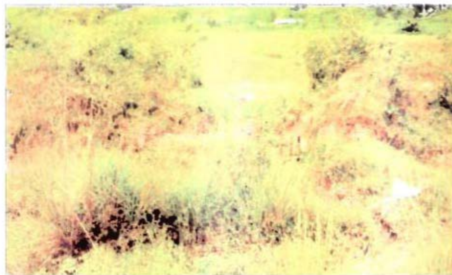
Thoubal Multipurpose Project – Manipur : Siltation, shrubs/weeds in Canal (MANIPUR)
