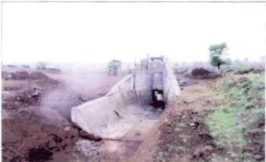
Canal work in progress in Kadakpurna River Project (MAHARASHTRA)
