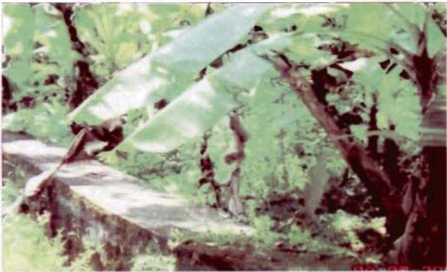
Pulamon Distributory of Kallada Irrigation Project – Canal filled with grass and plantations on the banks (KERALA)
