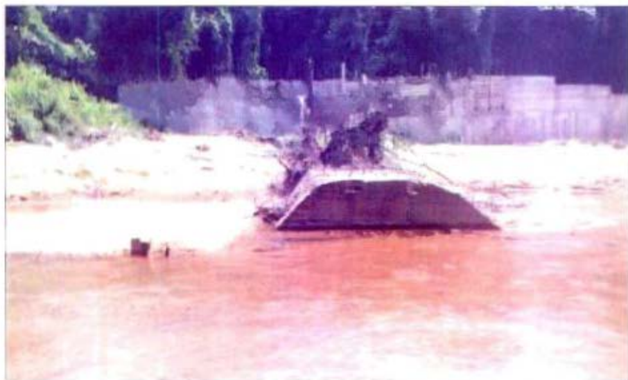
Ringdee MI Project—Headwork in progress (MEGHALAYA)
