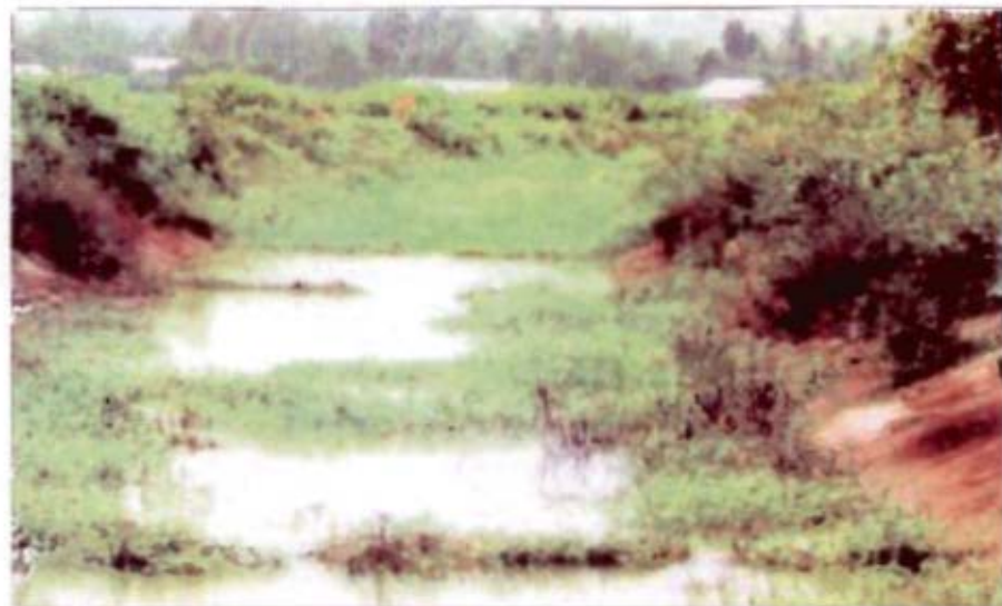
Thoubal Multipurpose Project—Siltation & shrubsweeds in canal (MANIPUR)
