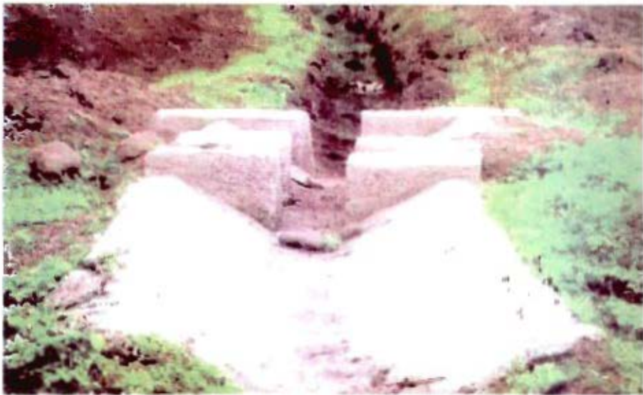
Slow progress of canal works in Arunawati River Project (MAHARASHTRA)
