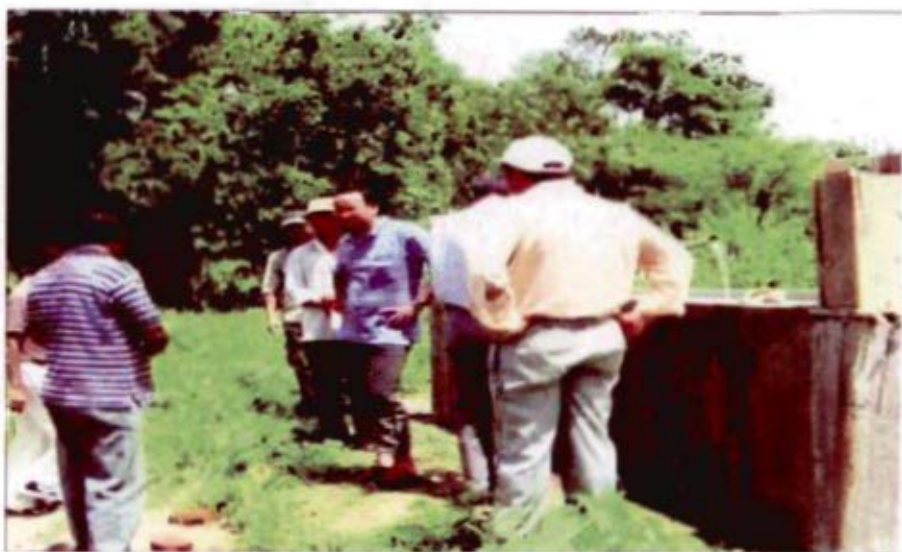
Reservoir under construction in Saihapui MI Project under Kolasib division (MIZORAM)
