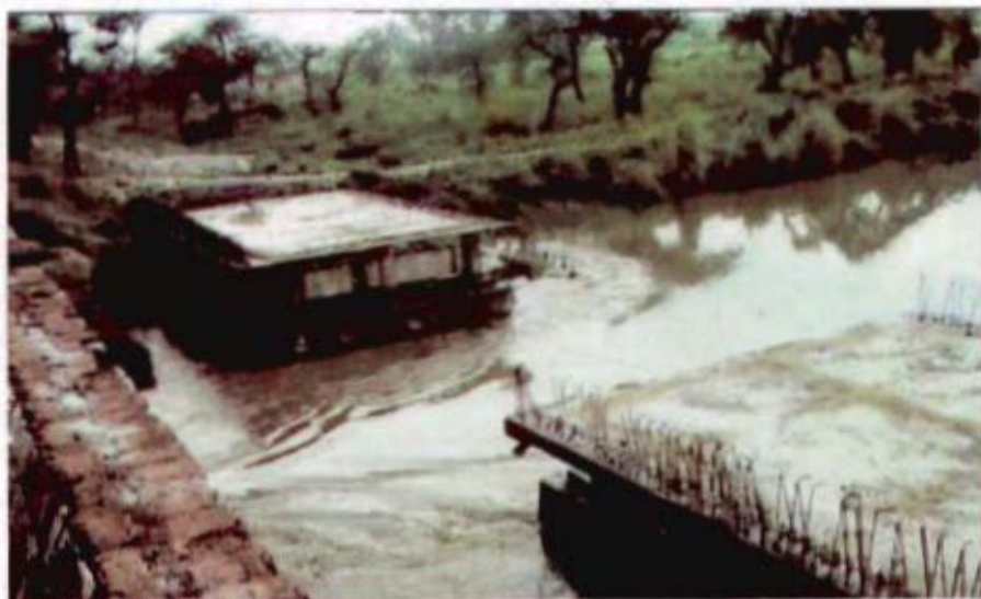
Agra Canal Project (UTTAR PRADESH)
